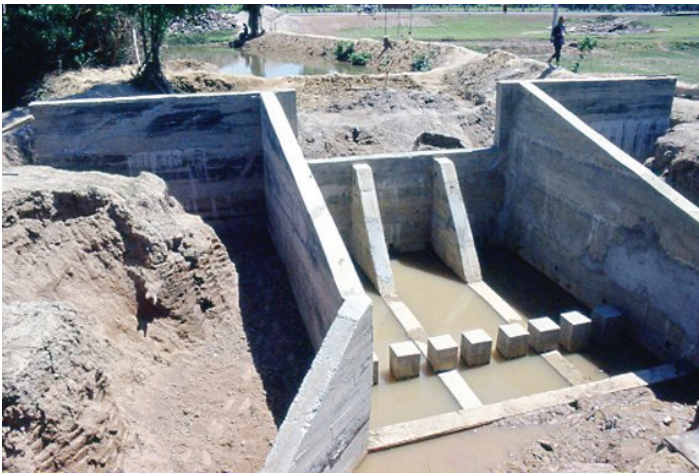
Spillway project nearing completion, May, 1981. Backfilling remains to be done.
